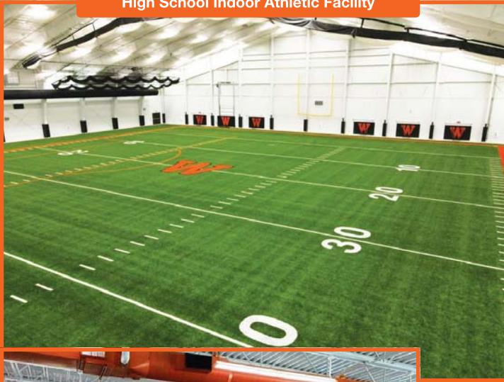
High School Indoor Athletic Facility
